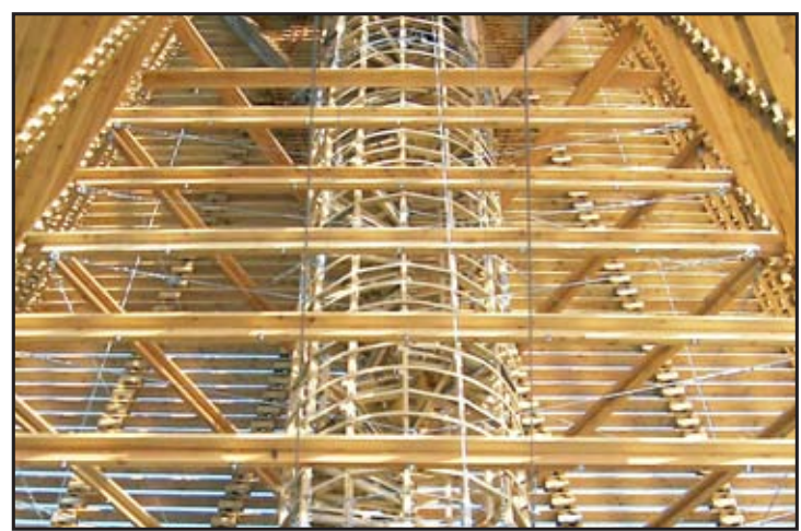
TOWER BARA I CHRUDIM C Z 2 0 0 9
