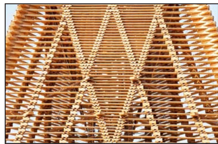
TOWER BARA I CHRUDIM C Z 2 0 1 1
