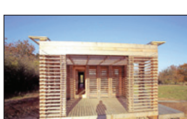
stack-house in slavicích C22007
